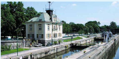
Lock chamber Štvanice
